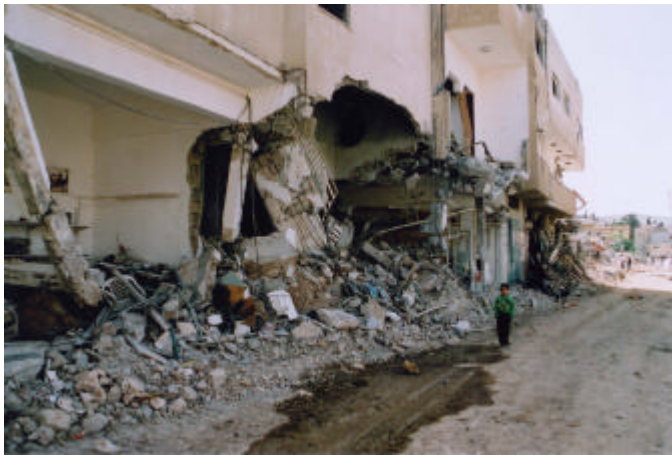
House frontages destroyed by tanks in Jenin refugee camp © AI
